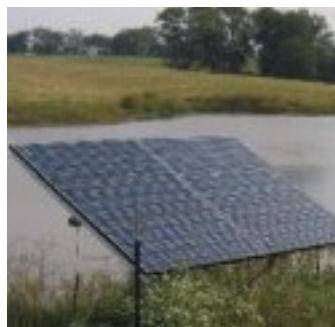
Paddock waterer fed by pond water pumped using PV panels (l).
